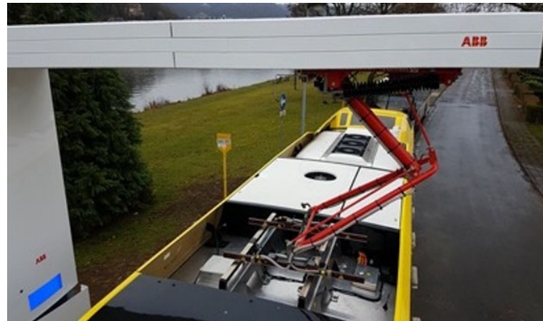
Overhead charger with pantograph (pantograph down)
